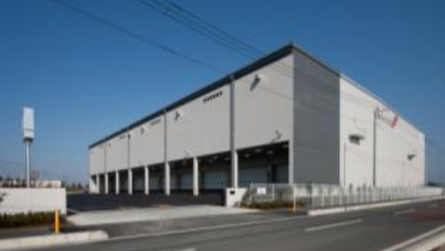
D Project Kawagoe Annex B
