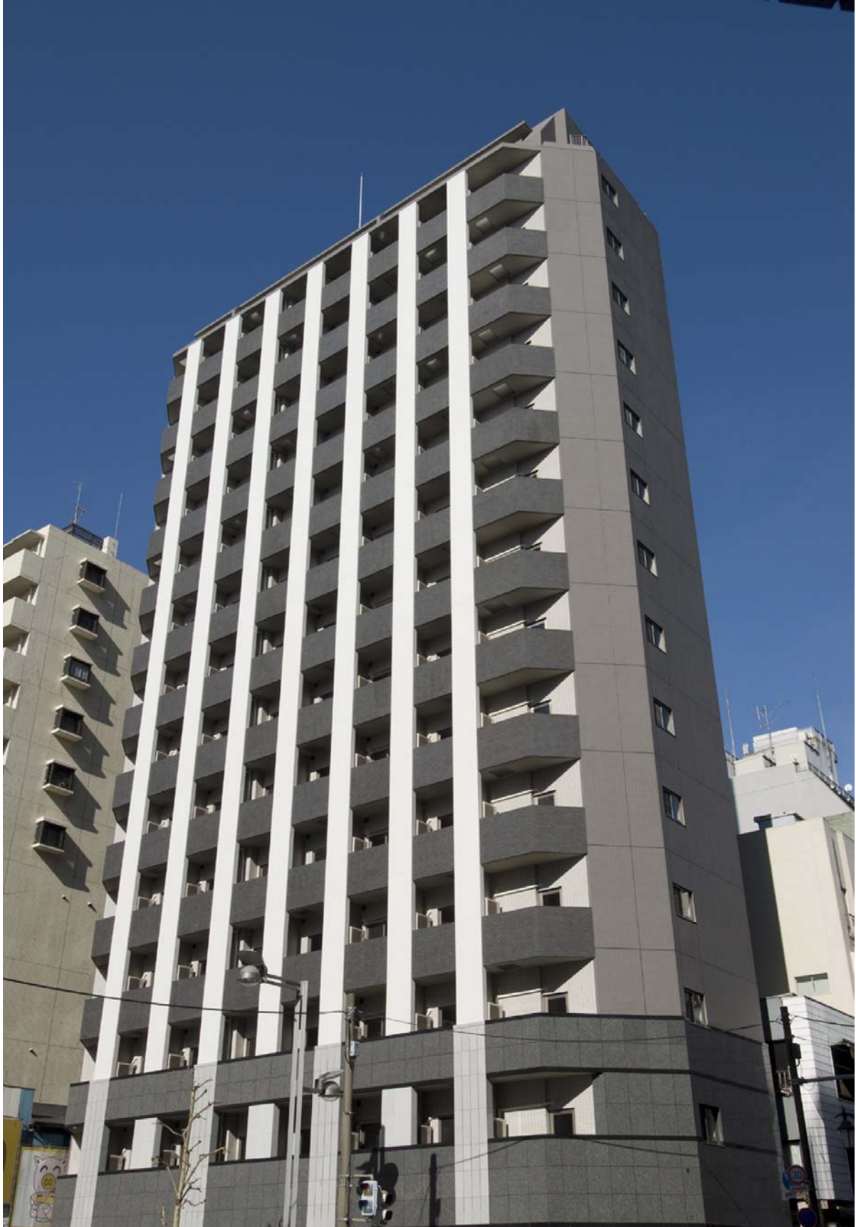
Photograph of the External Façade of the Property
