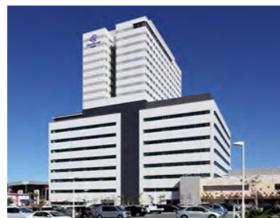
Naha Shin-Toshin Center Building (Daiwa Roynet Hotel Naha-Omoromachi) (Office, hotel and retail facilities)
