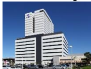
Naha Shin-Toshin Center Building
