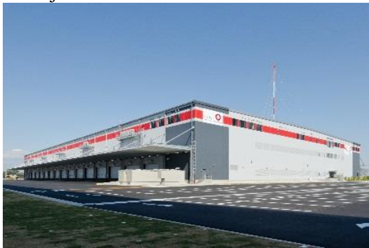
D Project Kuki II
